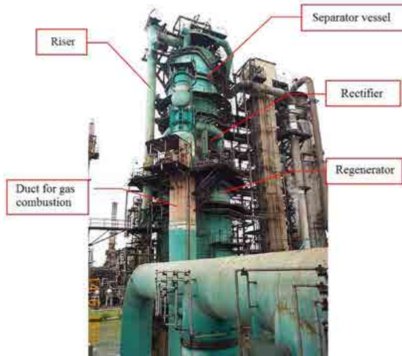
Figure 1.1: Converter set and ducts of the fluid catalytic cracking units. Source: MEDEIROS (2012).
