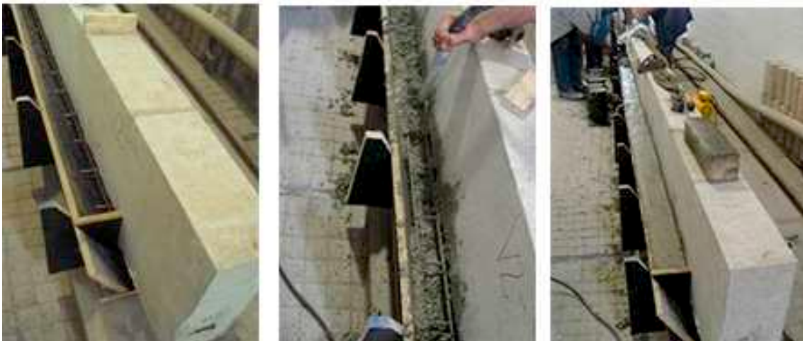
Figure B.1: Beam production phases. From left to right: first, the regular prismatic beam; the reinforcement casting procedure; and finally, the strengthened beam completed (courtesy of Vaz [123]).
